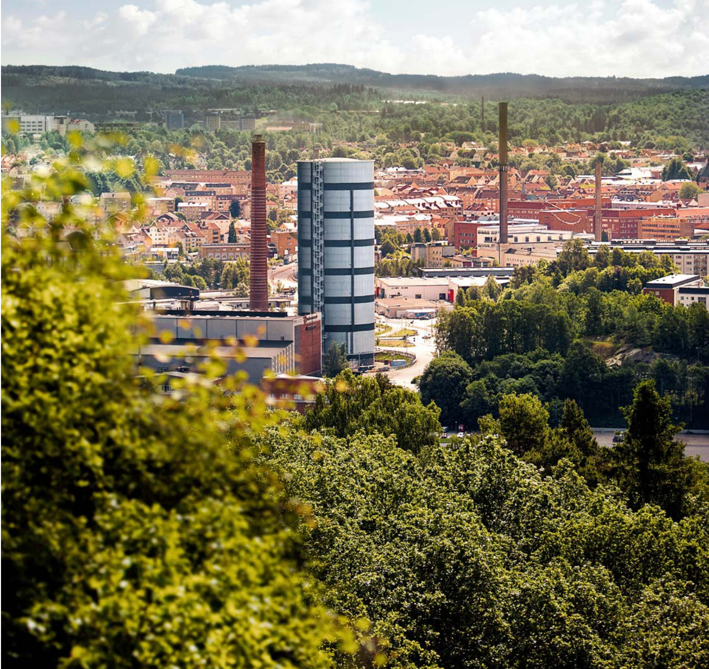
The thermal heat storage connected to the district heating grid of Borås is visible all over town.
