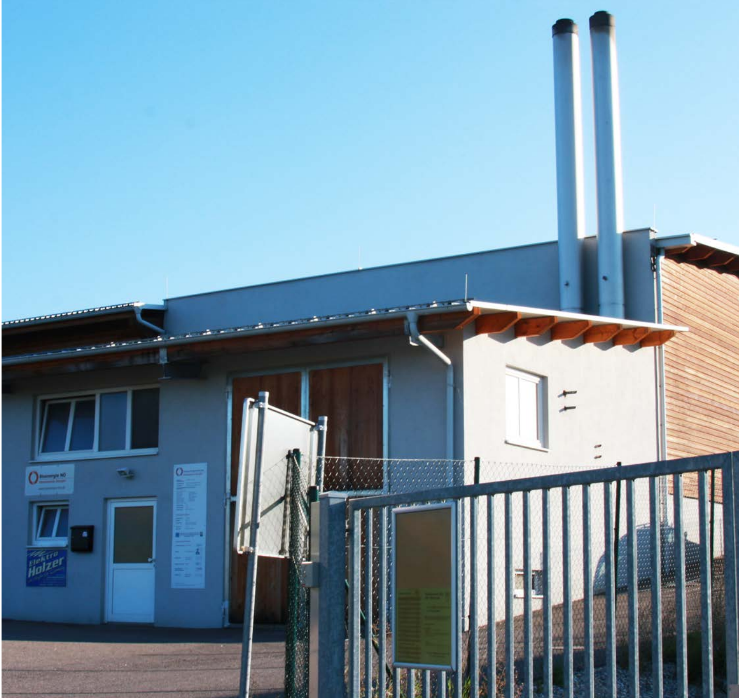
The district heating plant of Maria Laach is the smallest in the project and located in a rural area.
