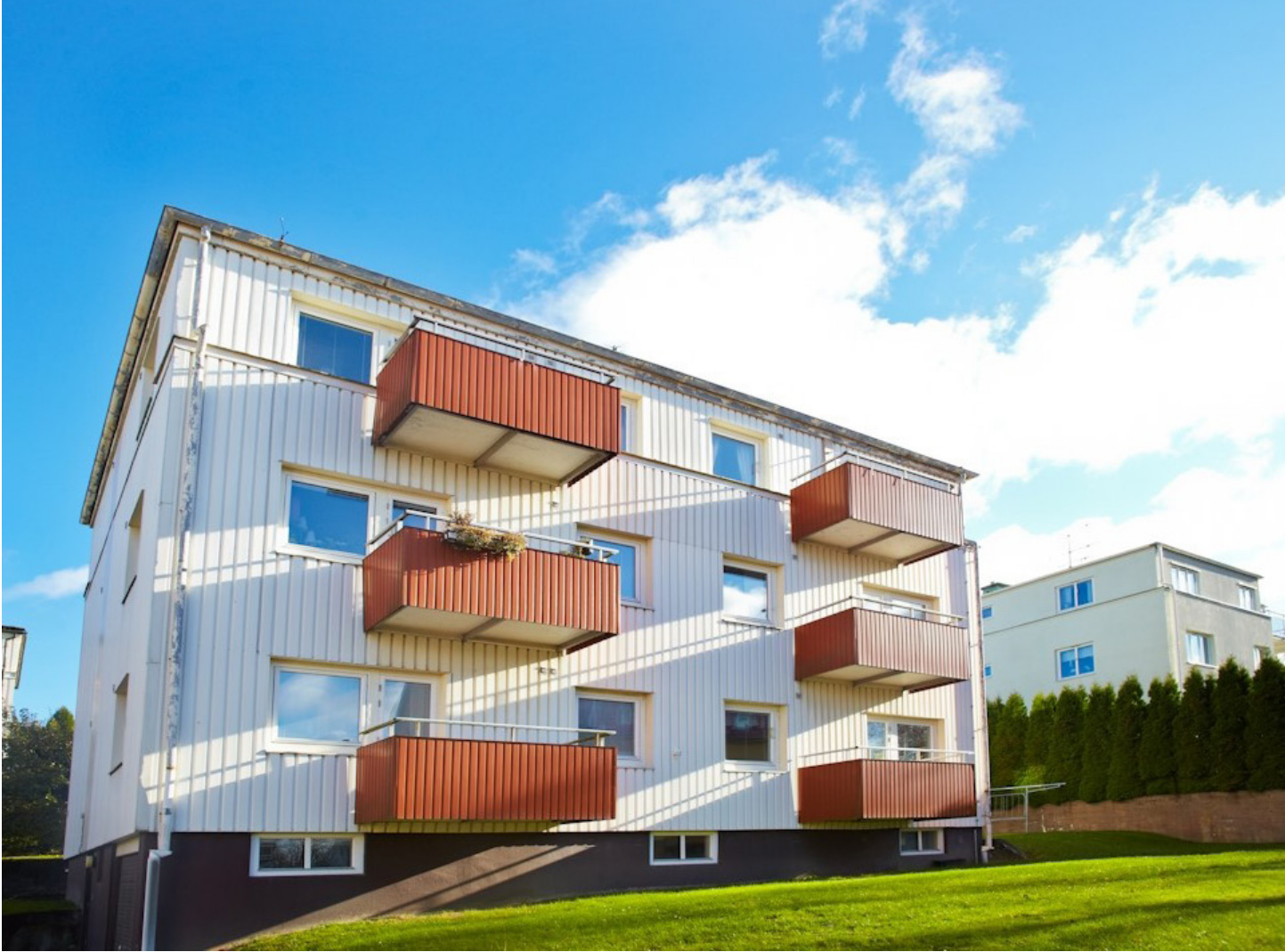
One of the houses in Borås where the solutions have been tested.
