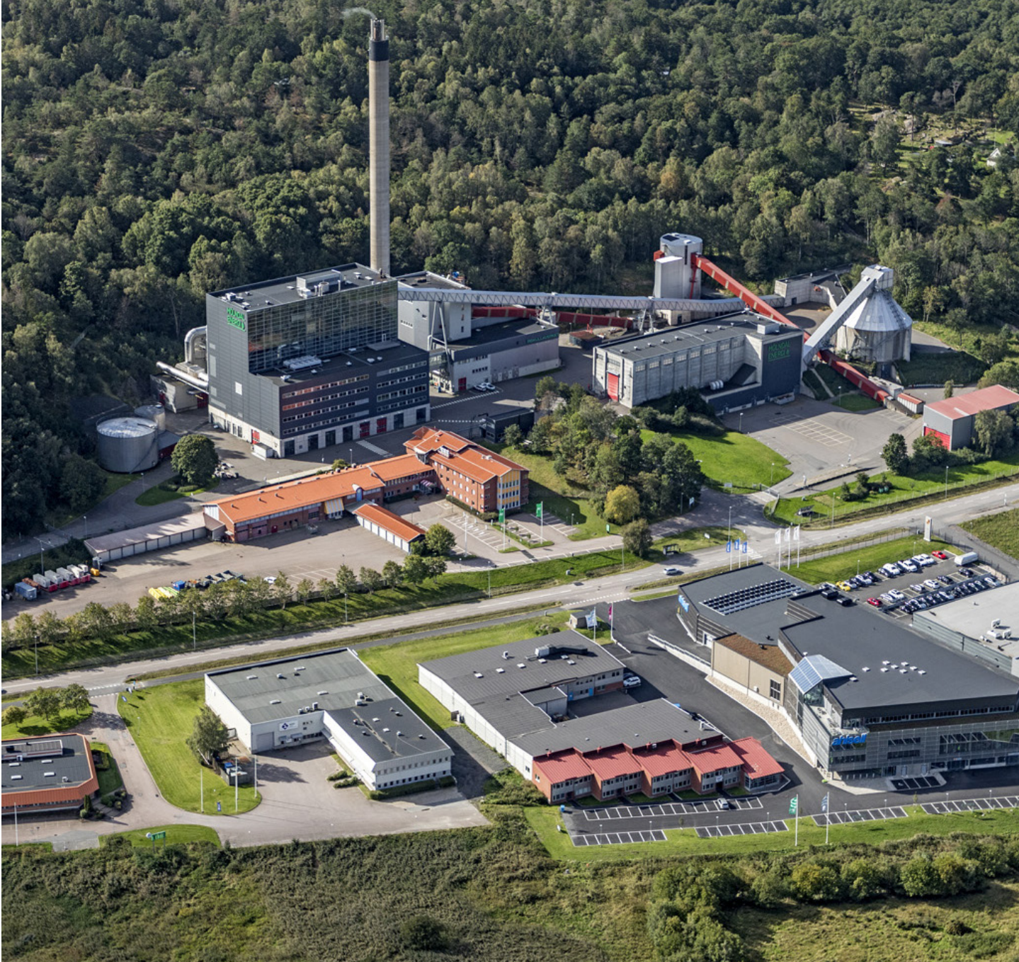
The district heating plant of Mölndal produces 290 GWh of heat each year.
