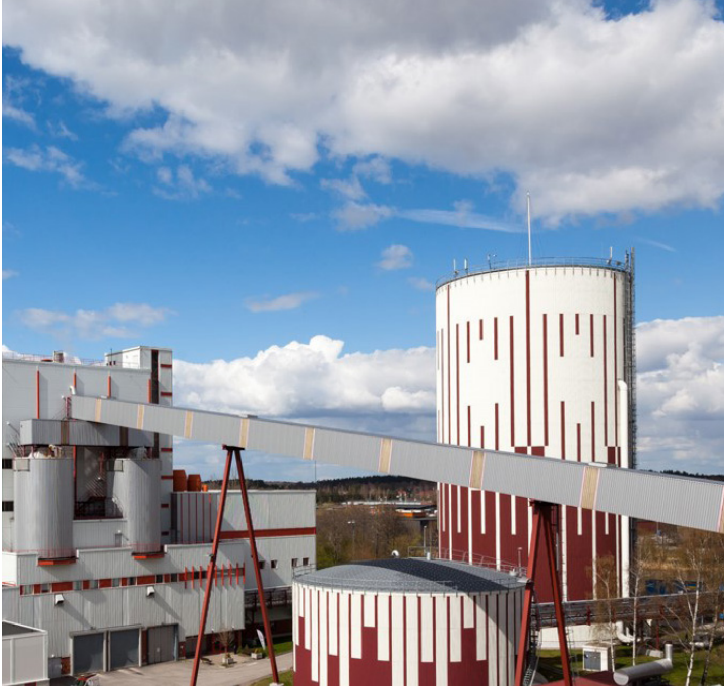
Eskilstuna's district heating plant with the characteristic white and red colours.
